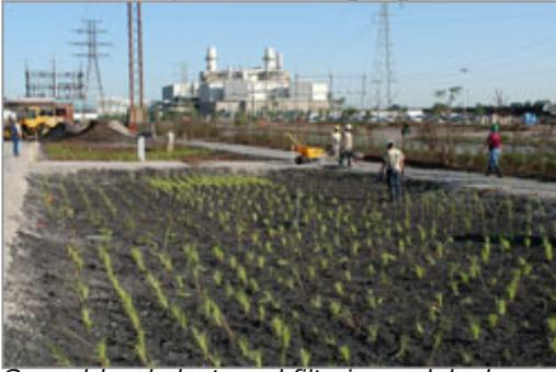
*Ground-level plants and filtering rock beds support the Dearborn Truck Plant's unique storm water management system.*
